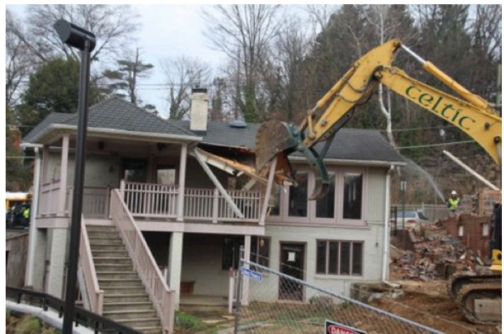
Demolition begins near the Lab School
