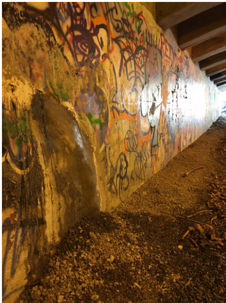
STINKY GRAFFITI: Lines show on March 24, 2019 along a crack patch in the tunnel under Canal Road at Glover Archbold National Park, where a sewage leak broke through in mid-March. Photo Credit: John Bray
