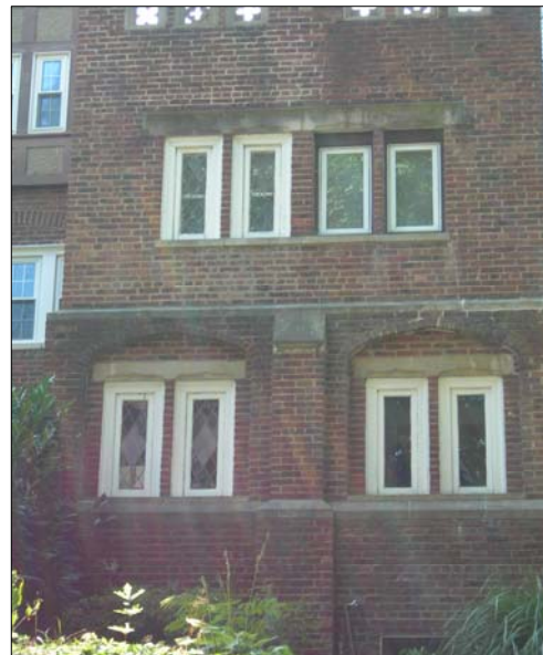
The replacement of historic windows with new windows that fail to match the details, configuration, and finish of the originals results in the loss of a significant architectural feature.
